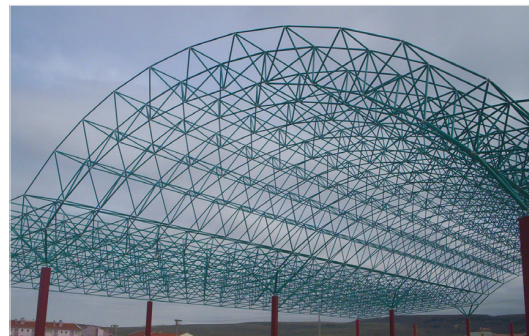
■ It may be used for steel construction manufacturing.
